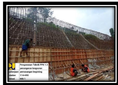
Gambar 10. Pekerjaan Retaining Walls
