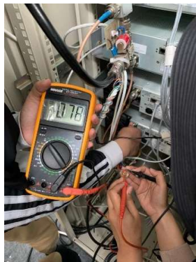
Gambar 11. Pengecekan Kabel Coaxial
