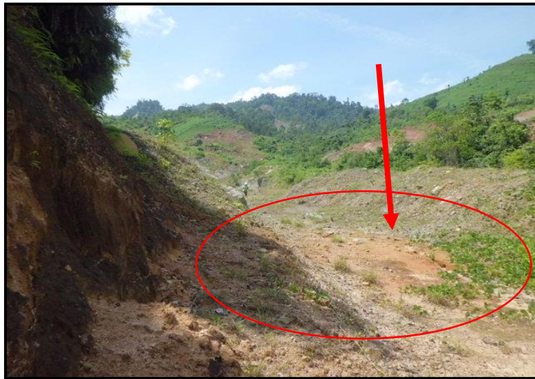
Gambar 6. Settling Pond Blok II pit 5
