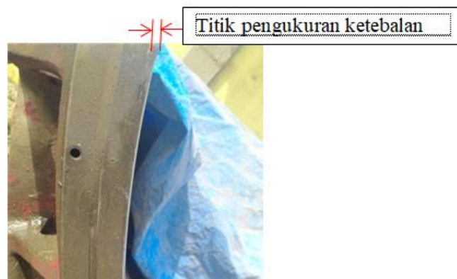
Gambar 6. Pengukuran Ketebalan Slide Shoe Bearing
