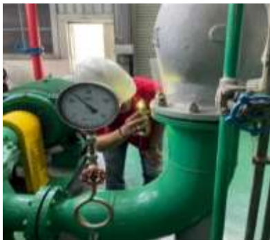
Gambar 9. Check Packing Gasket
