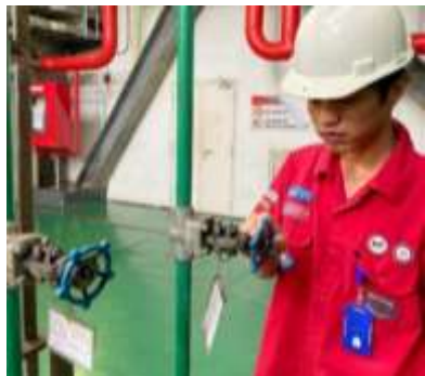
Gambar 10. Grease Manual Valve
