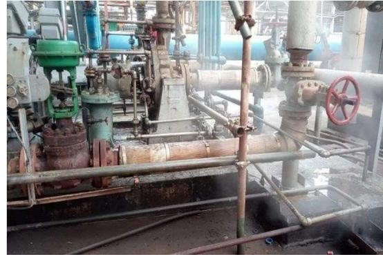
Gambar 5. Pompa Sentrifugal G-31-41-A
