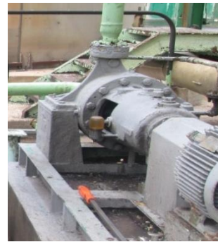
Gambar 6 Centrifugal Pumping Unit (CPU) [2]
